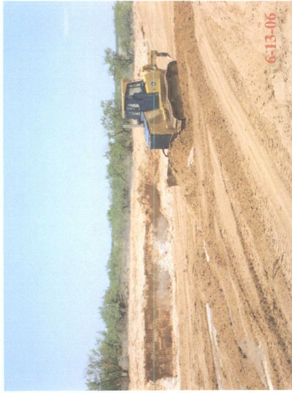
Dozer pushing backfill material into excavation at Test Point H
