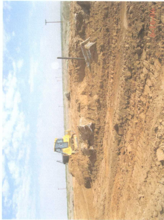
Dozer excavating contaminated soil at Humble State #3 well
