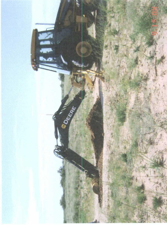
Excavation of delineation trench WL2.
