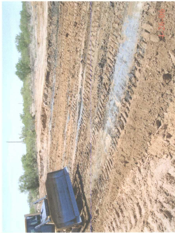
Dozer excavating contaminated soil at Test Point F at 2' deep
