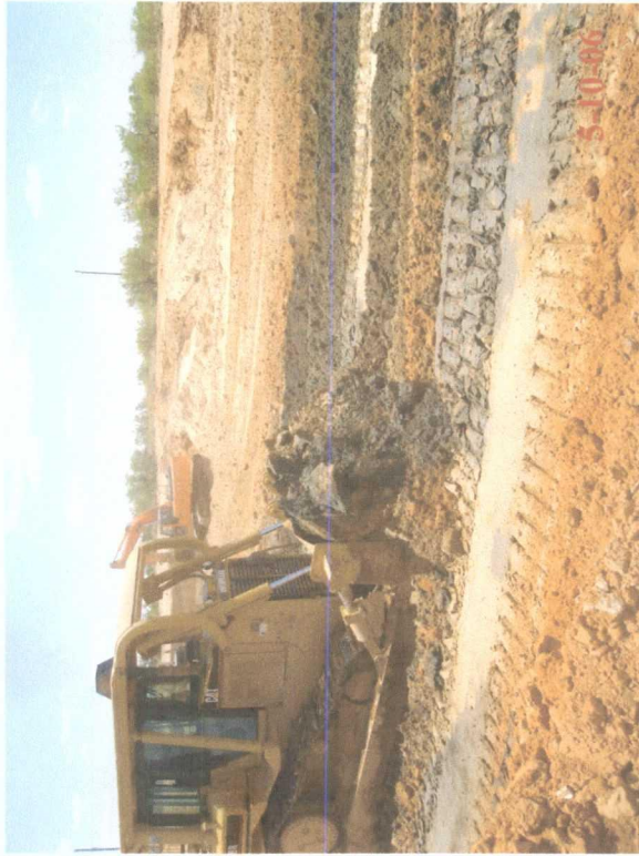
Dozer excavating contaminated soil at Test Point F at 6' deep
