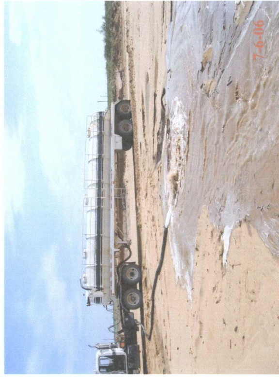
Water truck unloading fresh water for compaction
