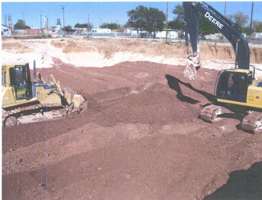
Photograph 9: Second Lift of Red Bed Clay
