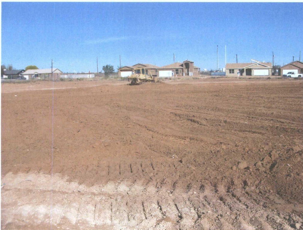
Photograph 12: Spreading Topsoil to Level Site
