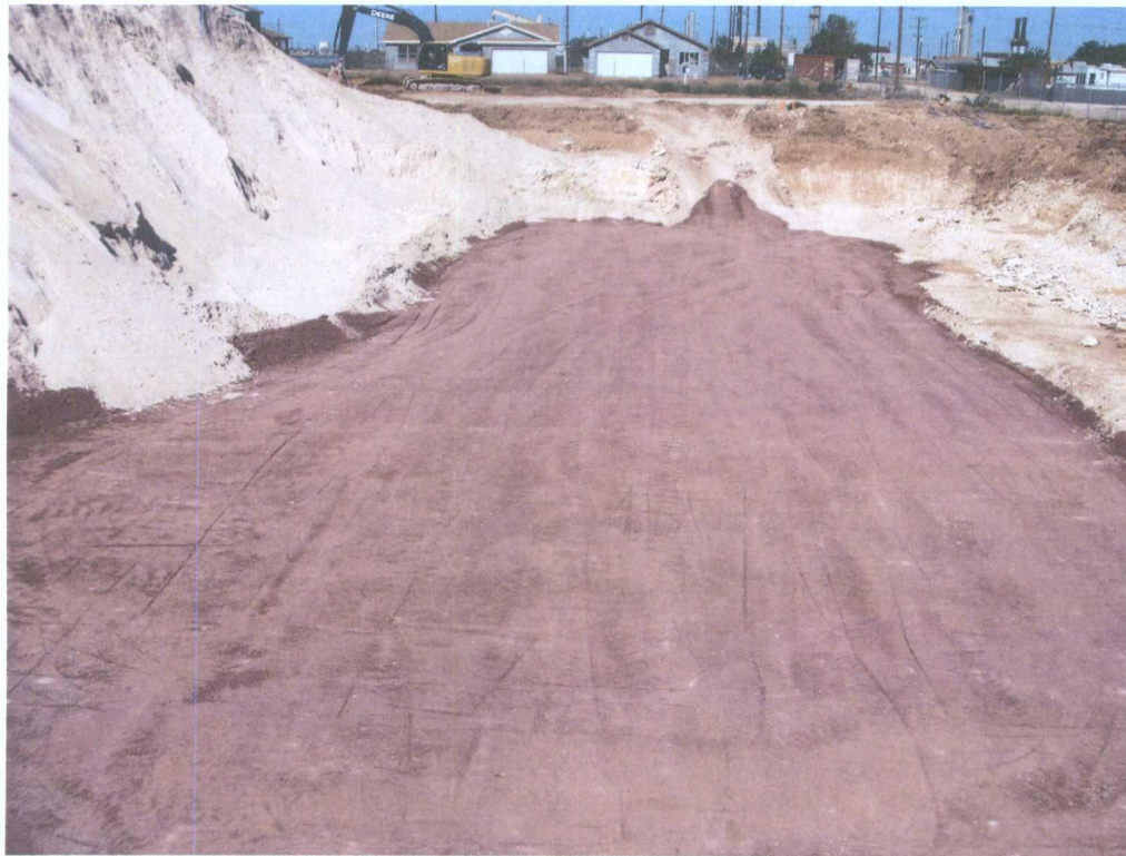
Photograph 8: First Lift of Red Bed Clay After Compaction
