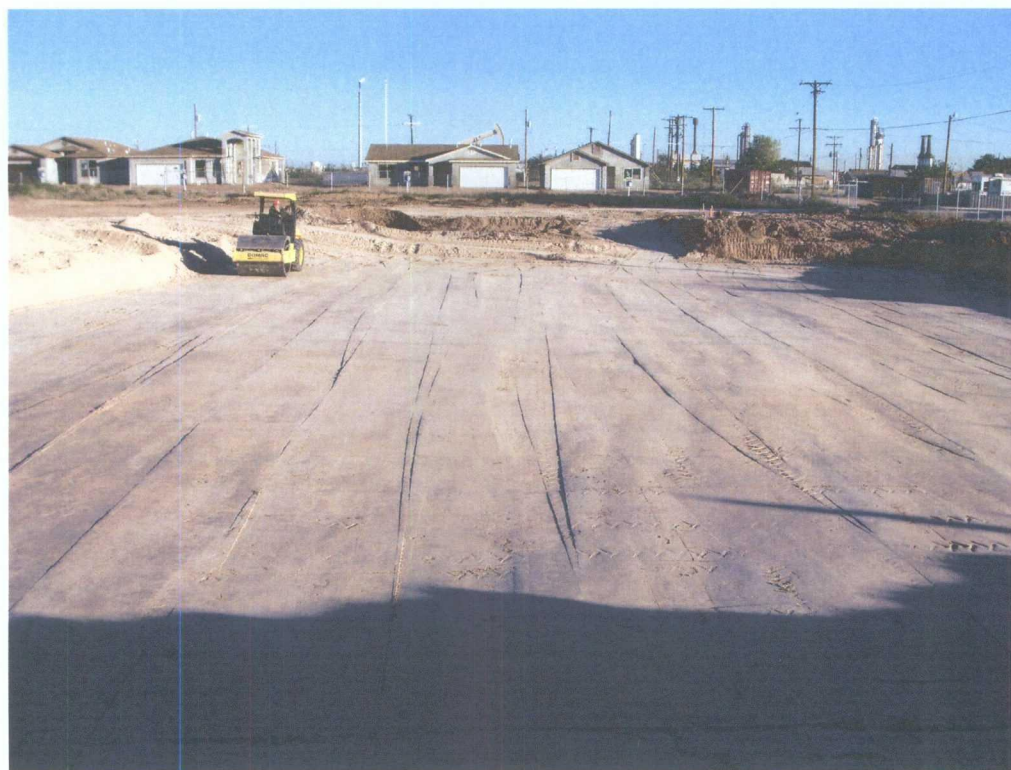
Photograph 10: Crusher Fines Covering Red Bed Clay
