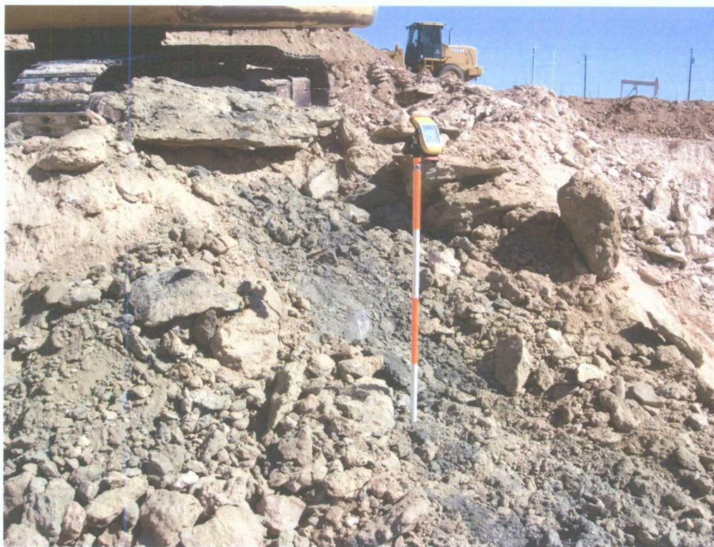
Photograph 4: Close-up of Hydrocarbon-Contaminated Soil, East Side of Excavation
