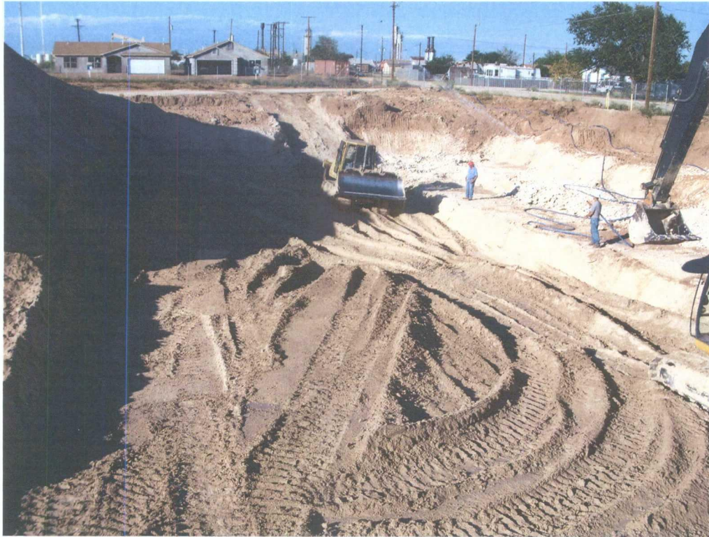
Photograph 7: Crusher Fines Placement in Bottom of Excavation
