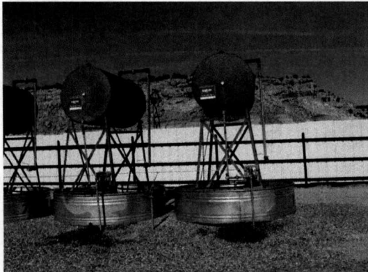
Photo 8: Discharge from saddle tanks.
