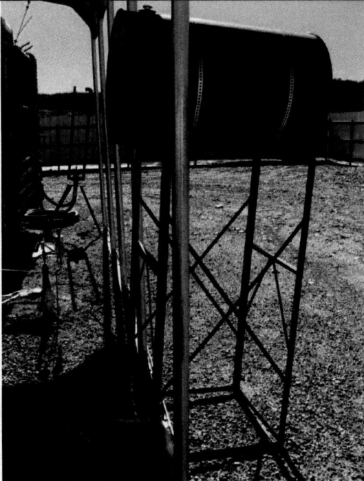
Photo 7: No secondary containment on saddle tank.
