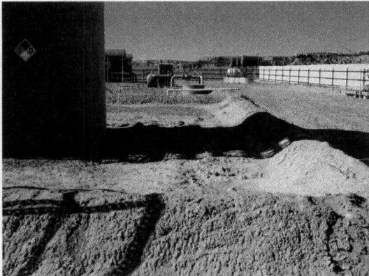
Photo 1: AST within bermed area.
