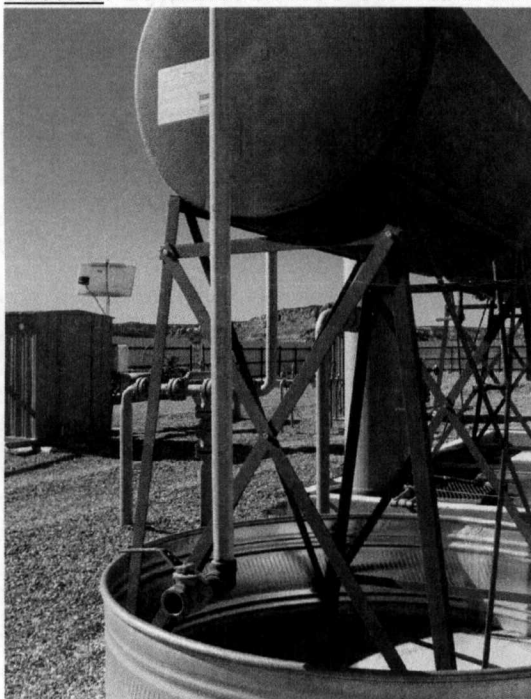
Photo 3: Saddle tank with protruding exit
