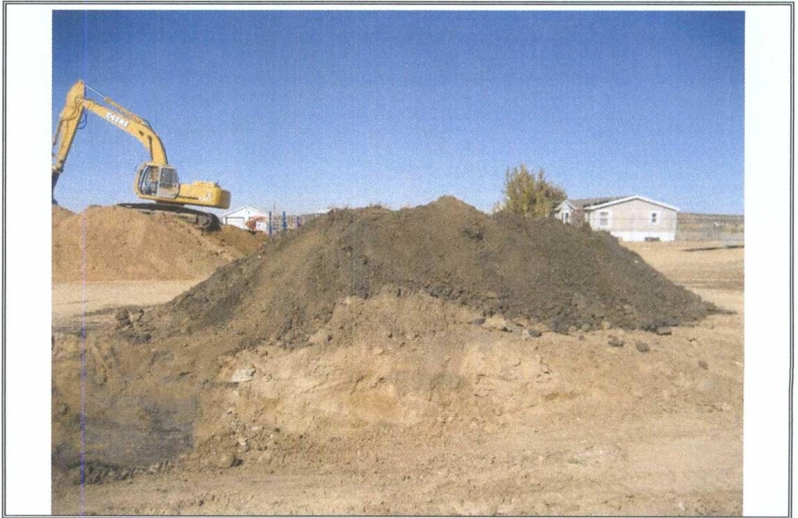
Photograph Number 11: View of contaminated soil staged for transport to TNT Land Farm.
