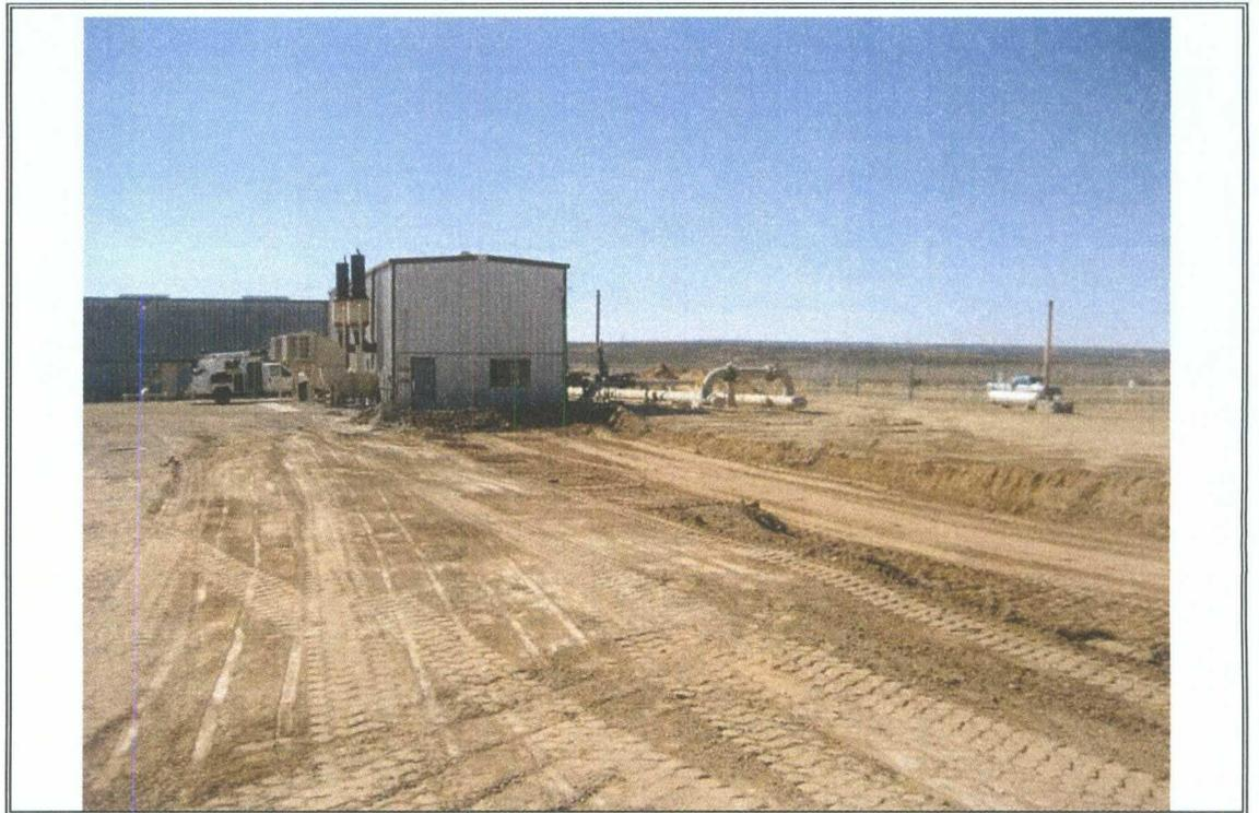
Photograph Number 13: View of the former Clark building in process of backfilling.
