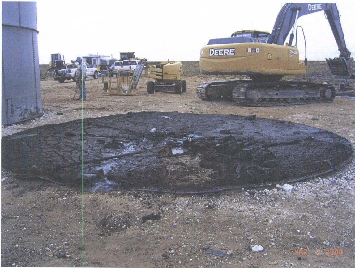
Exposed tank bottom at 1000 barrel tank T-2
