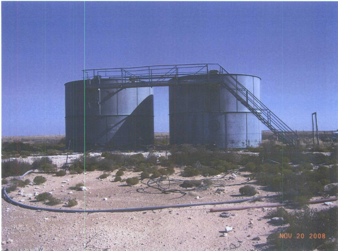
Figure 4- Two 500 barrel, steel, bolted tanks with catwalk.
