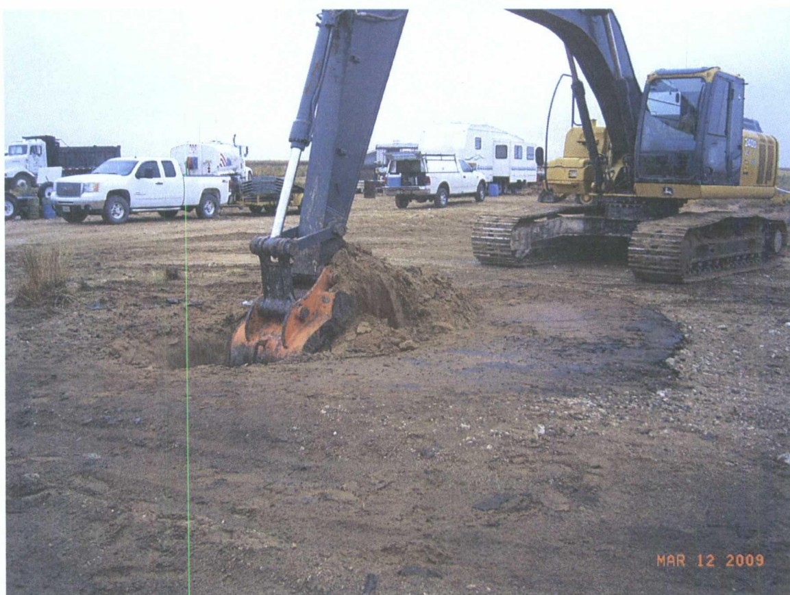
Beginning potholing of suspected contamination areas, T-1 tank battery location.
