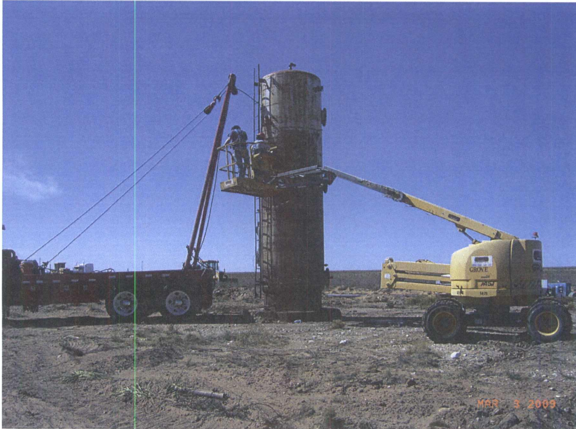
Decommissioning heater treater.
