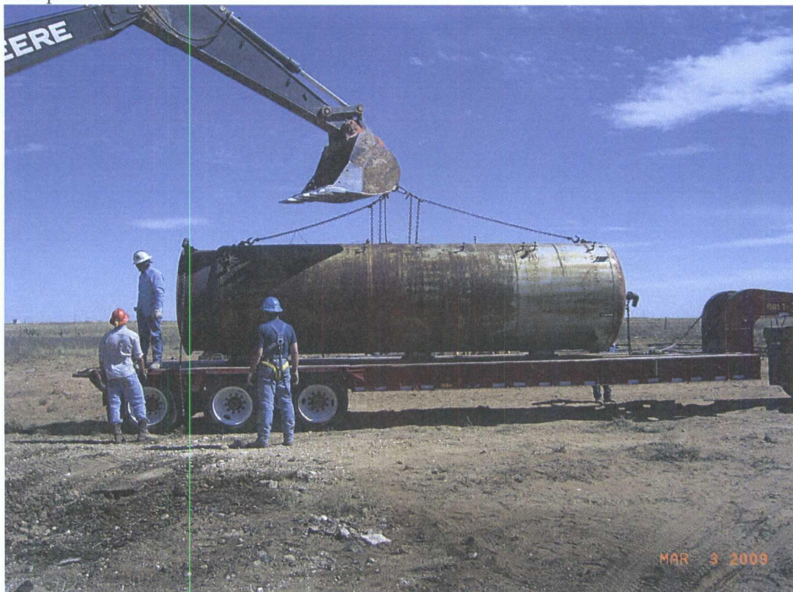
Securing heater treater for removal
