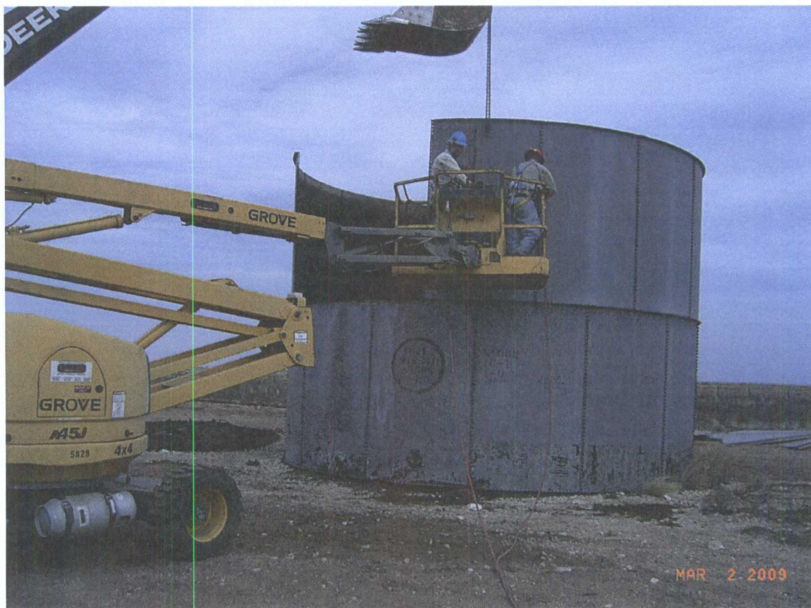
Unbolting panels at 1000 barrel tank T-1
