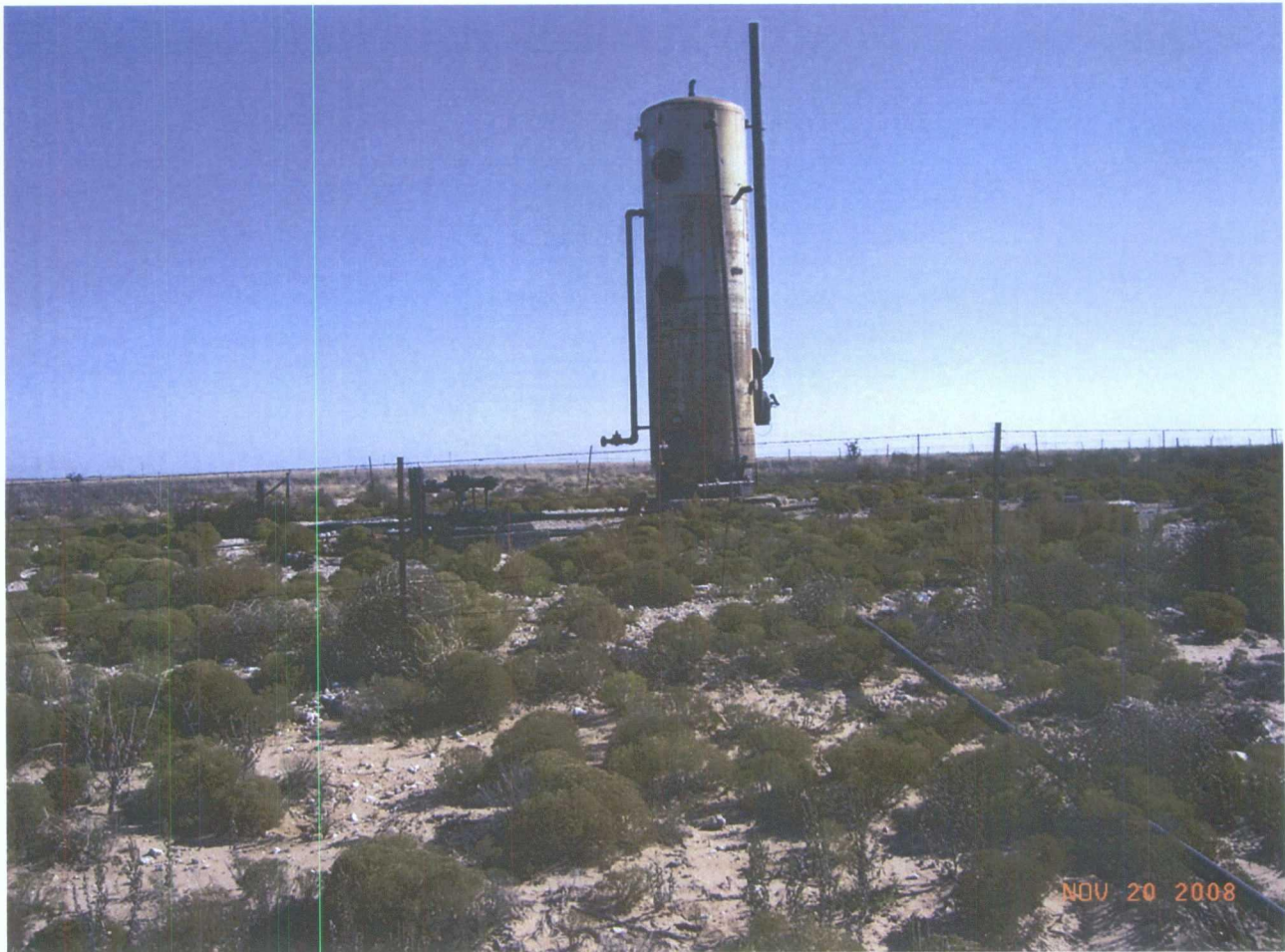
Figure 5- One 6' x 20' heater treater unit with manifold and piping.
