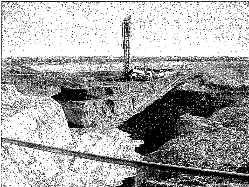
EK Queen Pearce 6-Inch Release Site, installing monitor well MW-3
