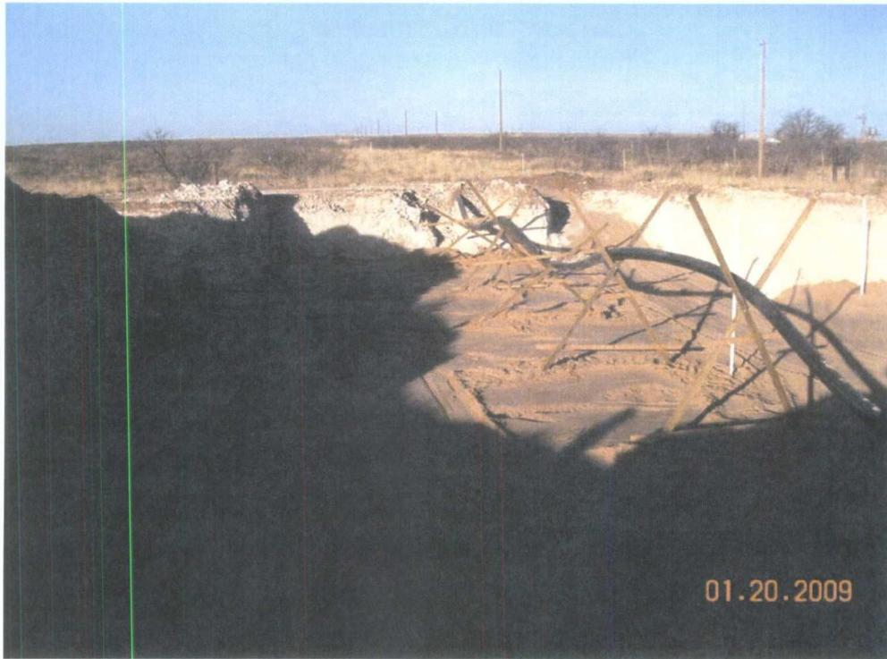
**Photograph No. 5 – Looking west at layer of cushion sand on bottom of excavation**
