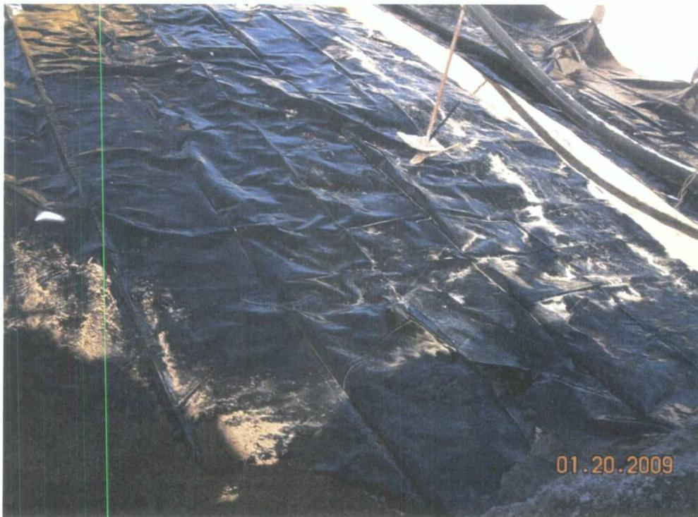
**Photograph No. 6 – Looking west a 40-mil polyethylene liner**
