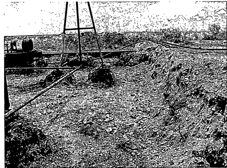
Site after excavation of impacted soil to hard rock at 2' to 3' bgs.
