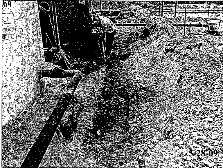
Excavation of impacted soil by hand around the tanks.
