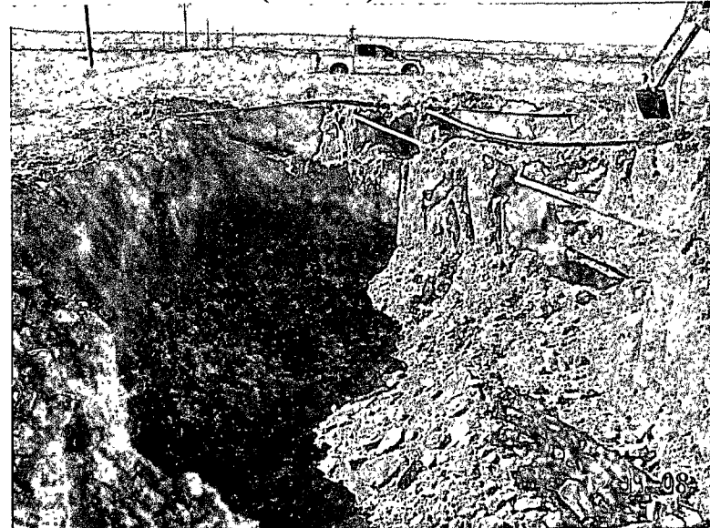
TP4 and TP5 after excavation of impacted soil.
