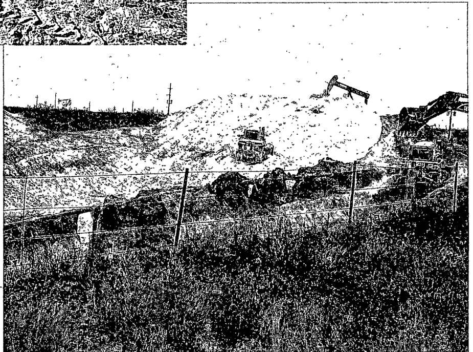
1/22/08 – Excavating and stockpiling soil for blending on surface. >
