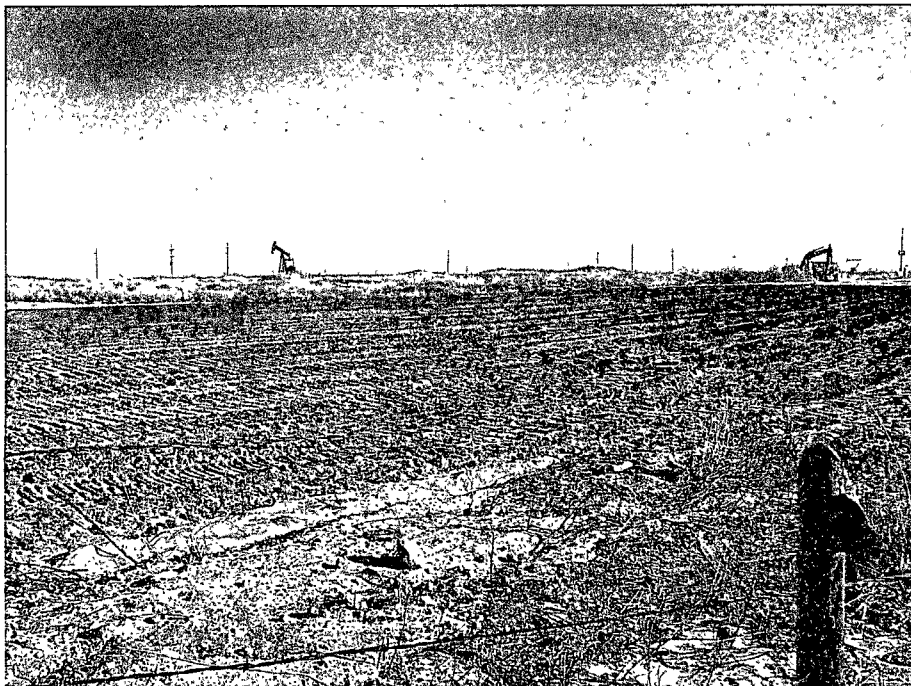
< 1/31/08 – Topsoil applied and location contoured.
