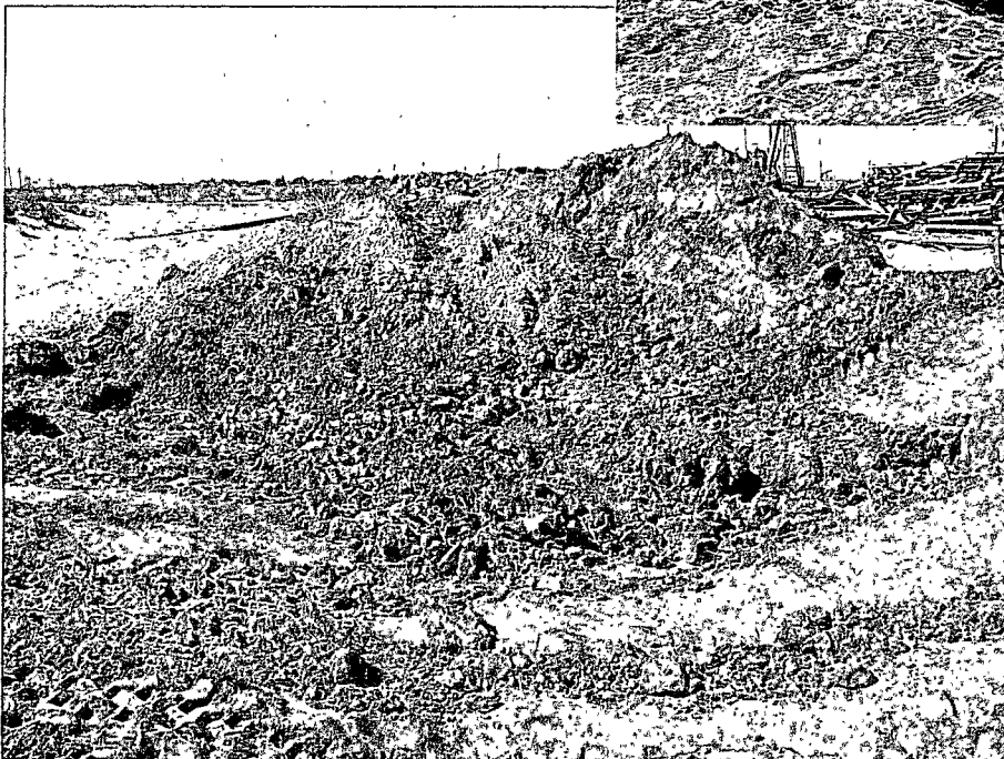
< 08/1/08 – Delineation trench in south portion of west release area. Note reduced iron sulfide.
