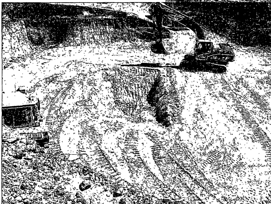
< 6/12/08 – Excavating from 25-ft bgs to 41-ft bgs to determine vertical extent of chloride contamination.
