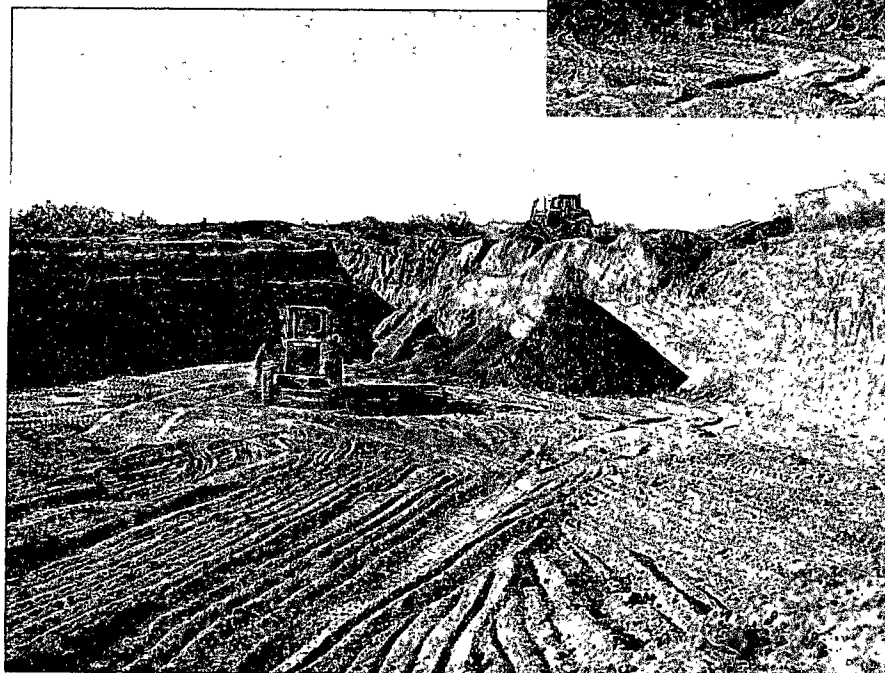
< 6/13/08 – Backfilling excavation with blended soil.
