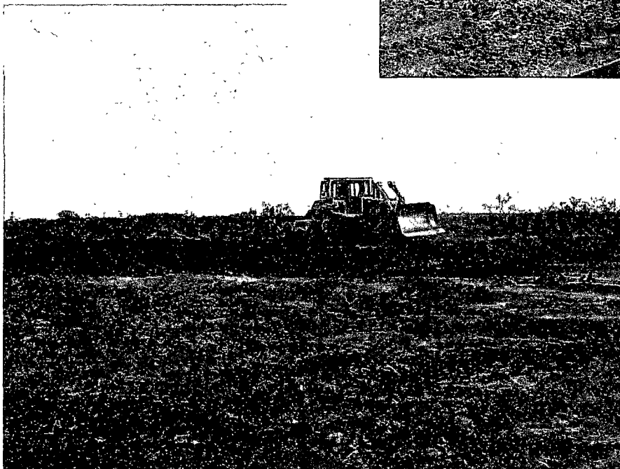
< 6/25/08 – Placing final 3-ft layer of topsoil
