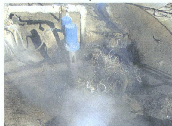
Housekeeping issue (debris in drain) evident along with cold weather conditions
