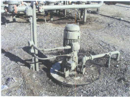
Soil staining around pump pushing fluids to tanks
