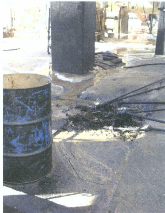
Housekeeping issue- debris in closed sump drain
