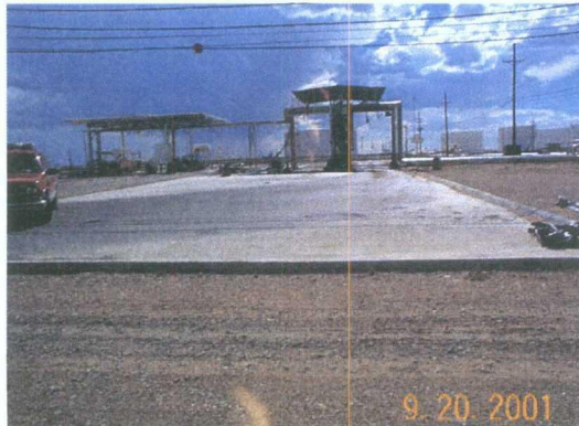
Chemical storage area w/ secondary containment
