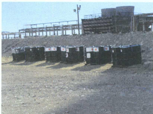
Drums (cleaner chemical) temporarily stored within bermed unlined area during Tk cleaning
