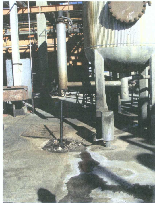
Drainage in the process area w/ route back to API Separator
