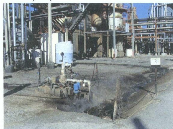
Closed sump storm water collection area w/ re-route to treatment system
