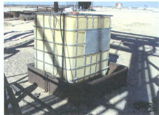
Chemical tote positioned over secondary containment
