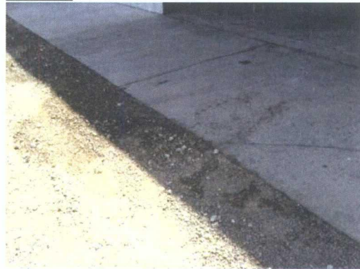
Photo 5: Wash bay area discharge on ground near entry/exit.
