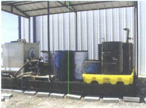
Photo 1: Fluid containment area.
