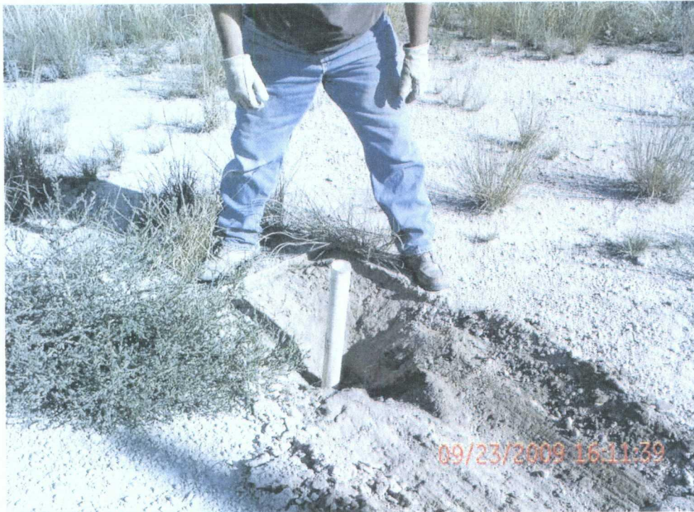
Plugging MW-1 at Hobbs E-32-1, NMOCD Case #1R428-65 9-23-09
