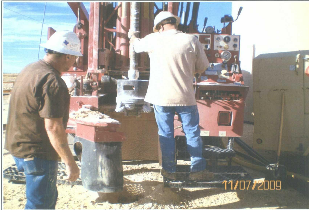
3. Installation of recovery well RW-2 at the brine well area (view to the south).
