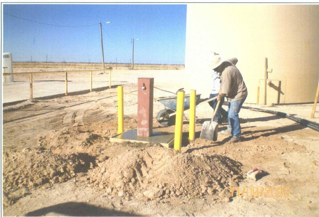
2. Completed recovery well RW-1 at the brine pond area (view to the north).
