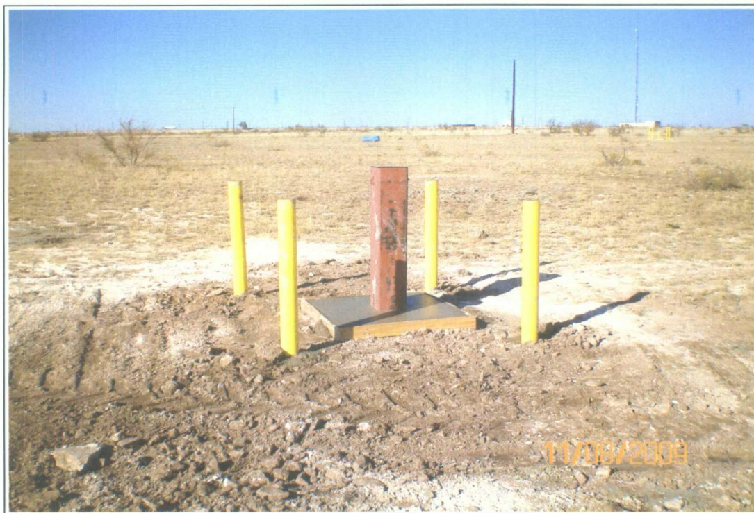
4. Completed recovery well RW-2 at the brine well area (view to the north).
