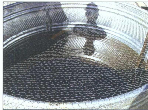
Photo 8: Remove fluids from secondary containment.
