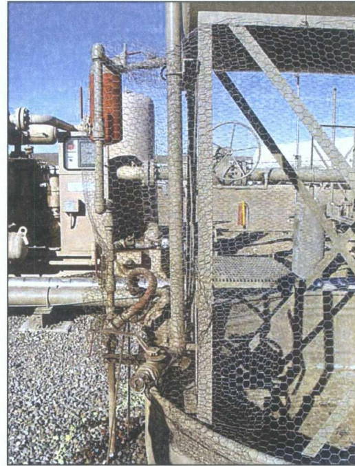
Photo 7: Remediate spill repipe load line to be within existing secondary containment or install a catch basin.
