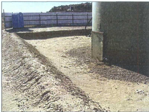
Photo 2: Earthen berm around AST. No immediate action required at this time.
