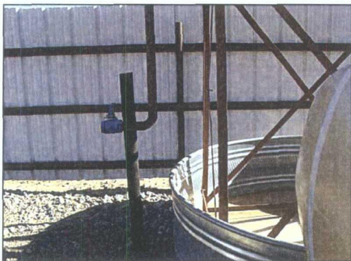
Photo 3: Repipe valve to be within existing secondary containment or install a catch basin. .
