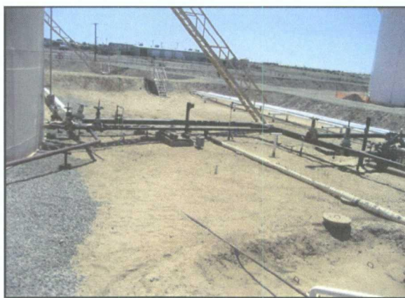
Clean up within Tank #29 Berm
