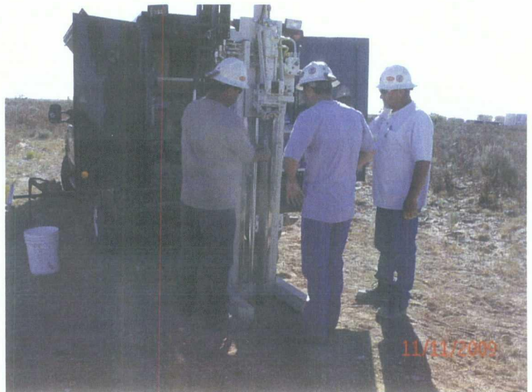
Installation of soil bores
