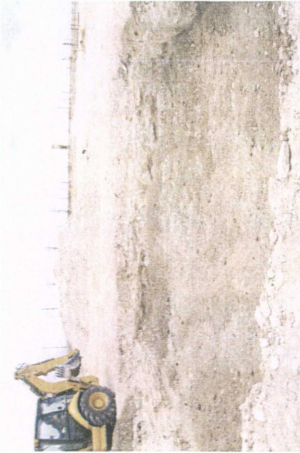
site backfilled up to 4' BGS in preparation for GCL
