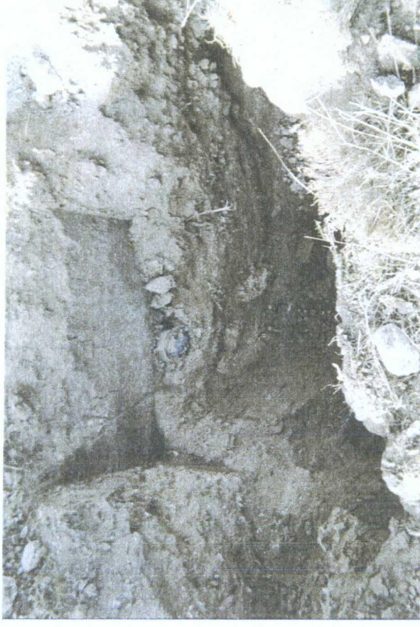
delineation trench at former junction site at 7' bgs
