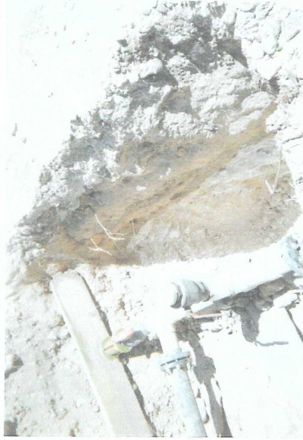
delineation trench to 7 ft BGS at former junction site
