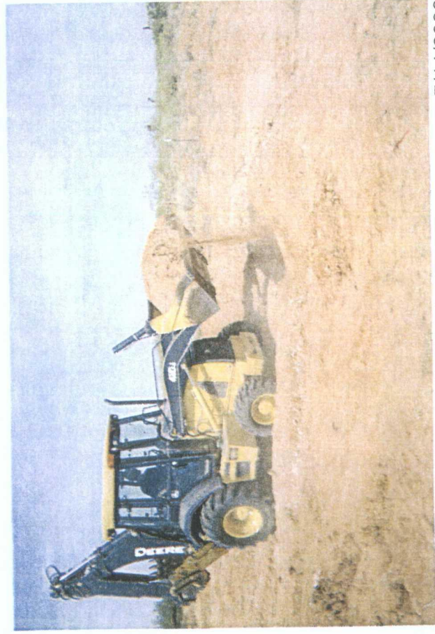
spreading clean, imported soil on site
