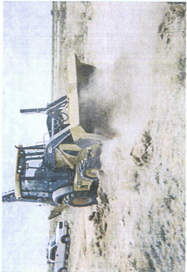
backfilling excavation
