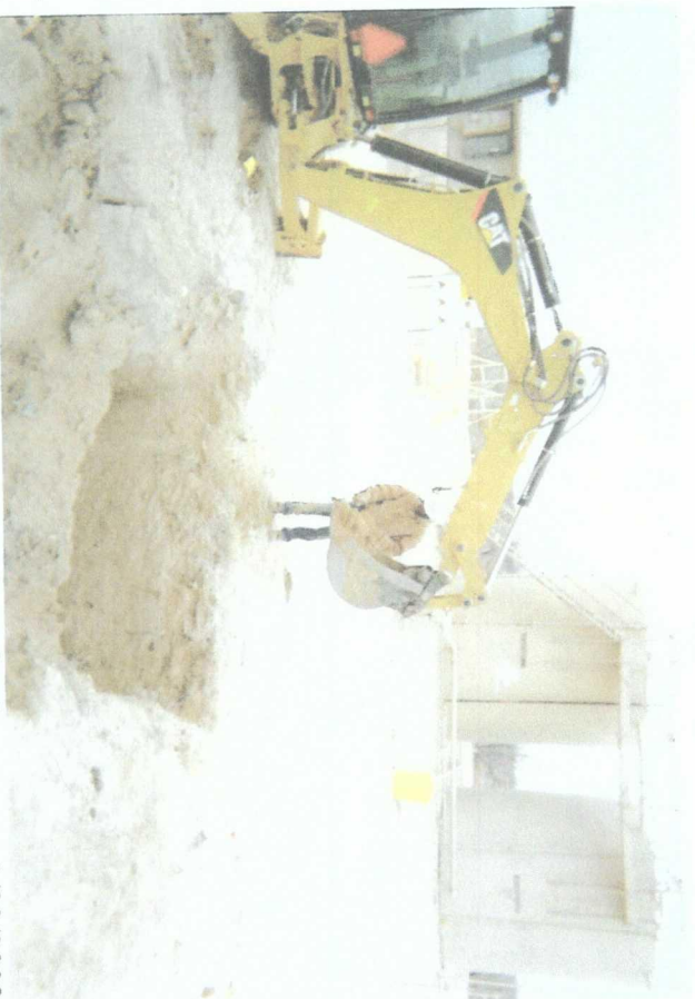
taking a sample of delineation trench 5 ft north of source 1/22/2008
