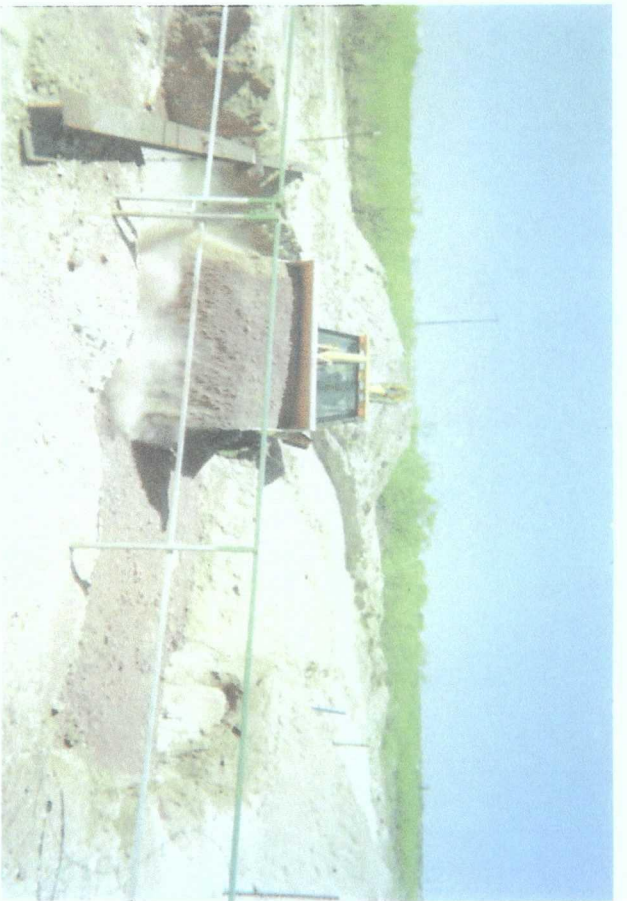
installing clay barrier
