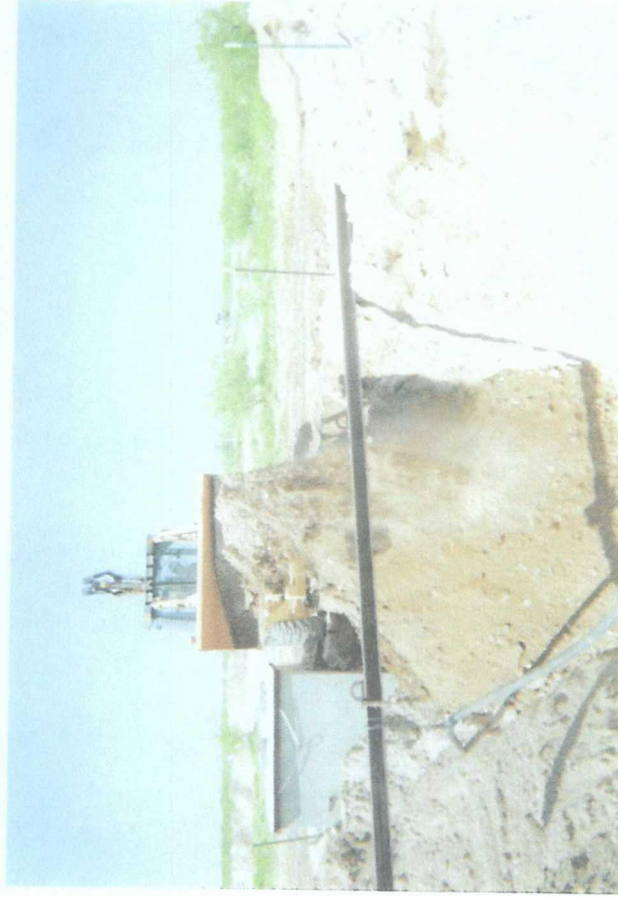
backfilling excavation up to 6 ft BGS
