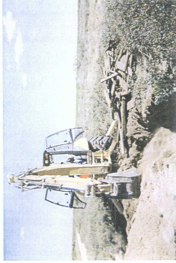
backfilling 5x3x12-ft-deep excavation
