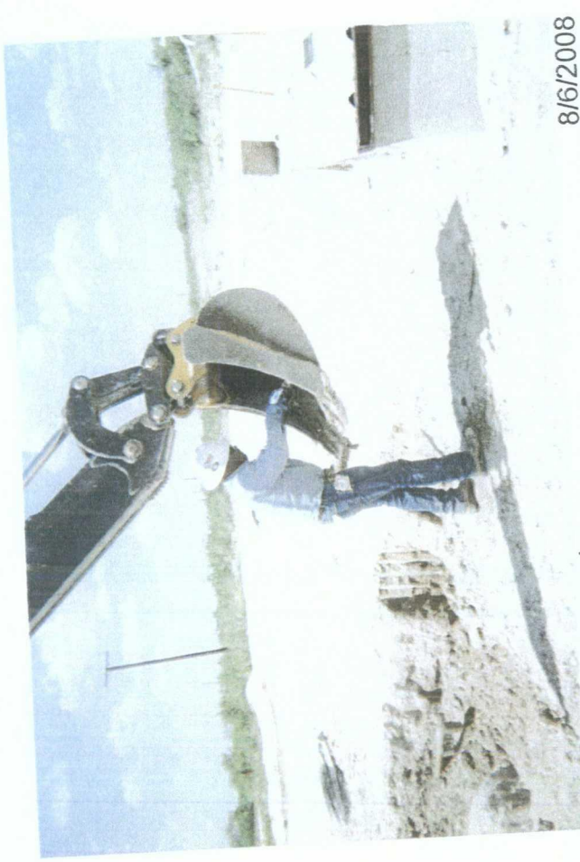
collecting a soil sample
