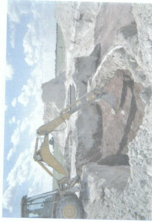
clay barrier being compacted
