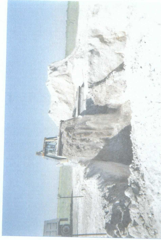
backfilling excavation site up to 5 ft BGS, facing west
