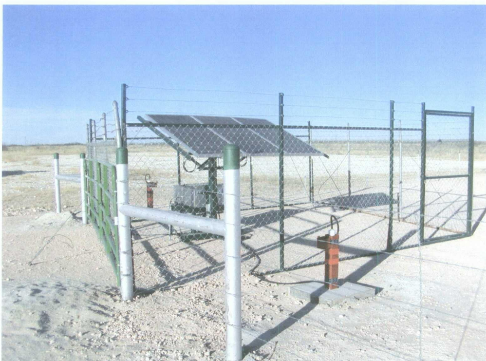
Figure 3a (above) – EME H-20 SWD solar powered bio-sparge system, view across system toward the southeast (in the direction of groundwater flow). Figure 3b (below) close-up view showing bio-sparge air injection wells looking toward the north.
