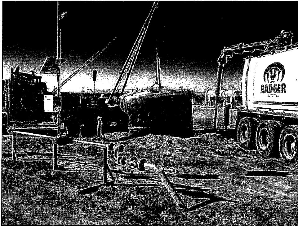
Tank being removed from its hold.
