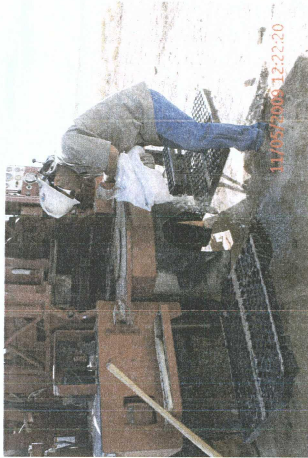
plugging SB #1 with bentonite
