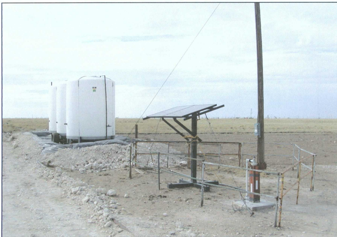
Figure 3 – Vac K-35-1 solar-powered groundwater recovery system.
