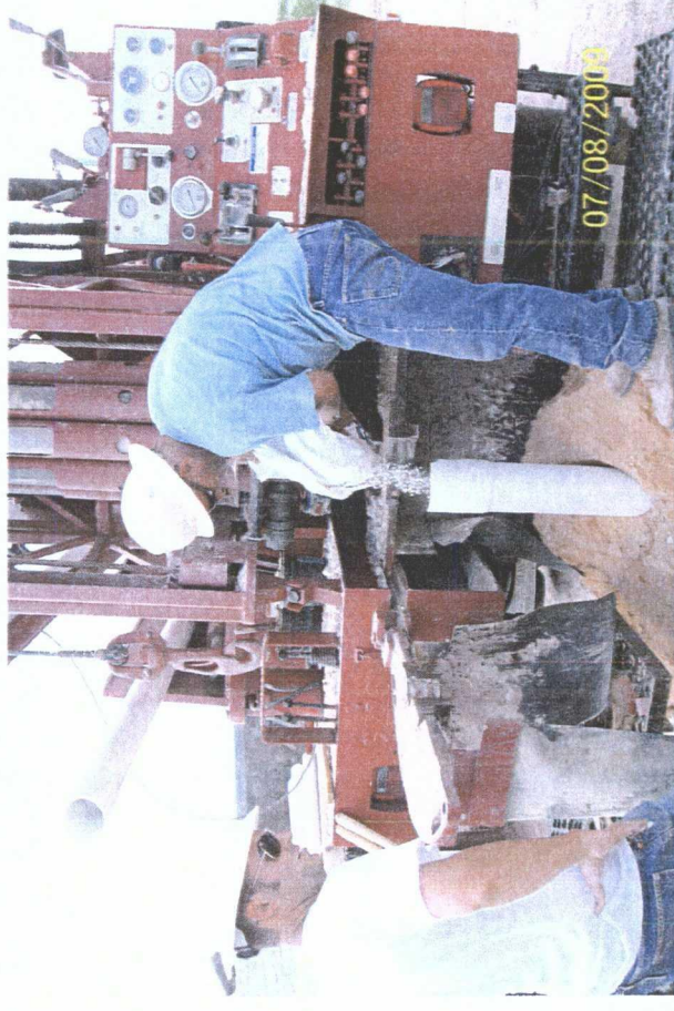
plugging SB #1 with bentonite
