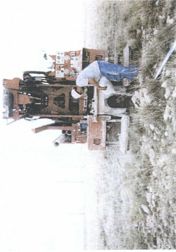
plugging SB #1 with bentonite
