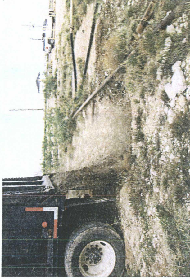
backfilling the excavation
