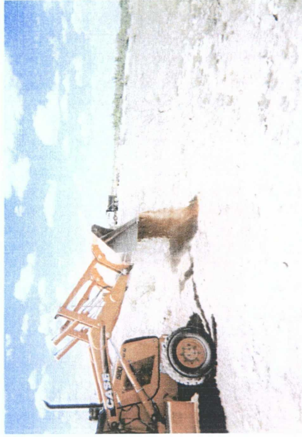
backfilling the former junction box site with clean soil
