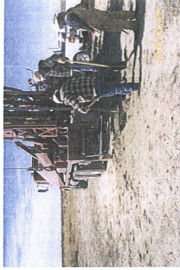
soil boring the former junction box site
