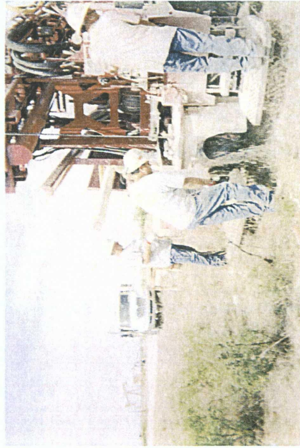
plugged SB #1 with bentonite
