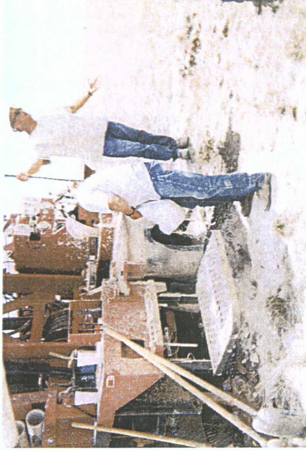
plugging SB #1 with bentonite
