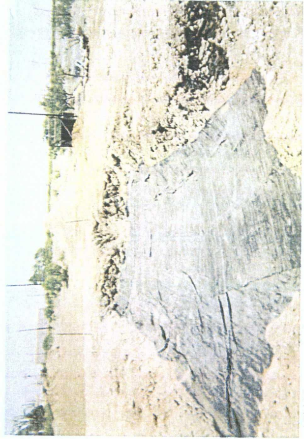
45X20 geosynthetic liner installed
