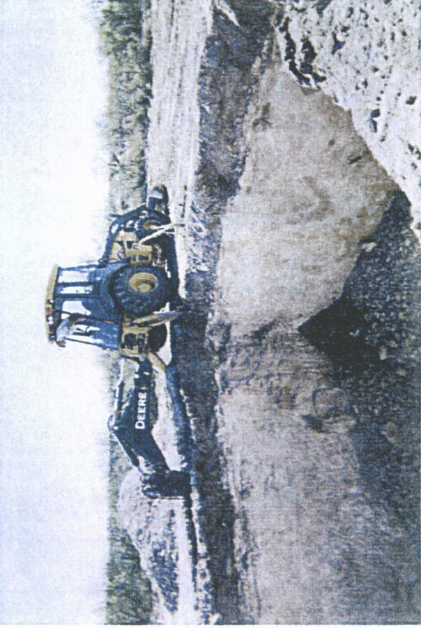
excavating former junction box site to 30x30x12-ft-deep, facing east
