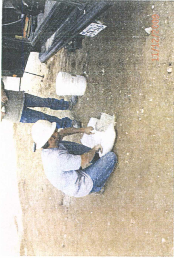
Plugging entire soil bore with bentonite
