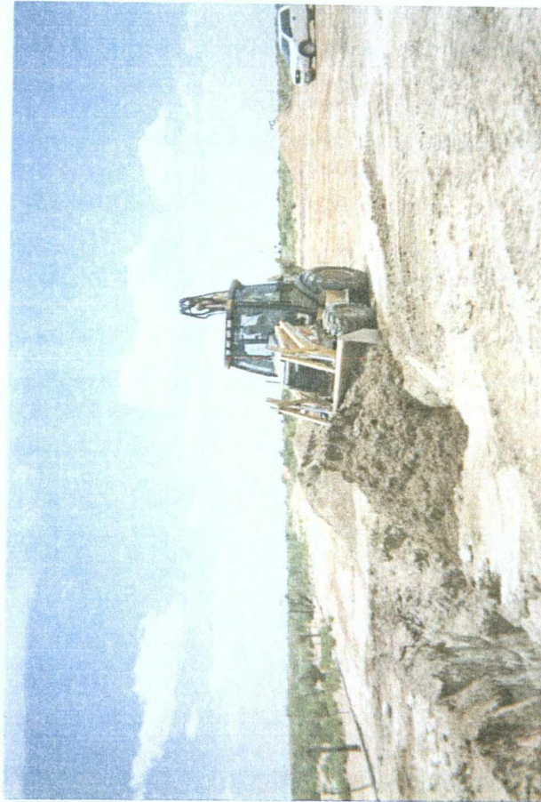
backfilling the excavation with clean, imported soil
