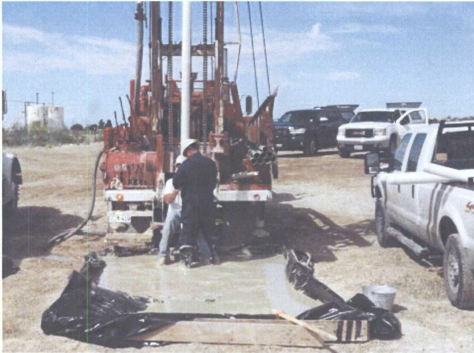
Installing Monitoring Well MW-14 Looking West
