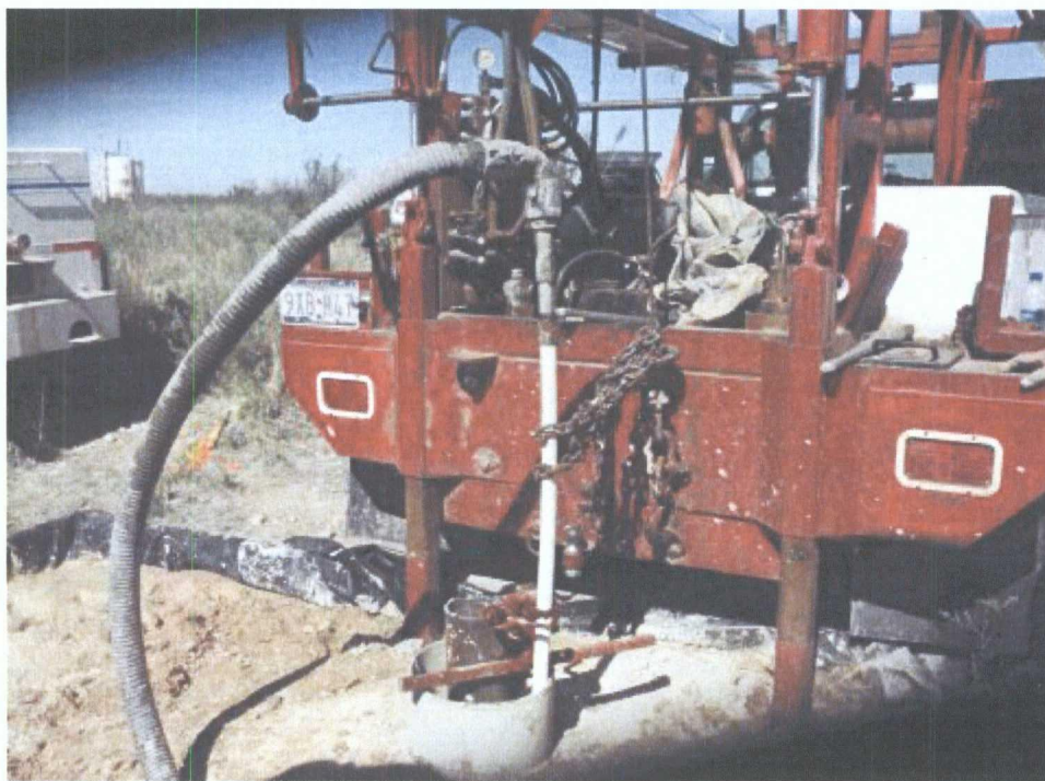
Grouting Conductor Casing at BH-9 Looking Southwest
