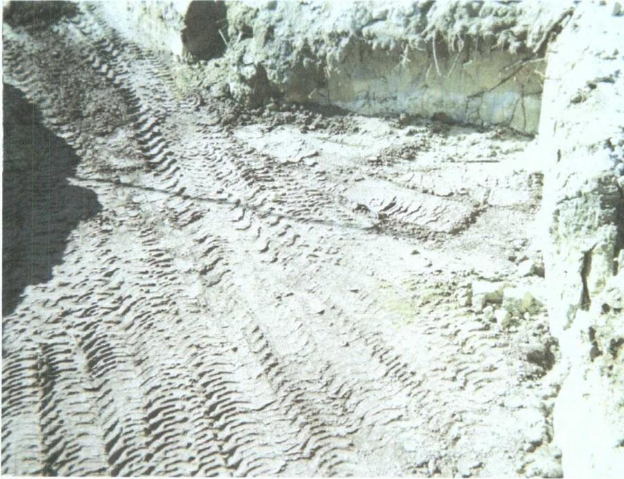
**Figure 4** – Clay infiltration barrier installed at EME N-18 boot in August, 2004.
