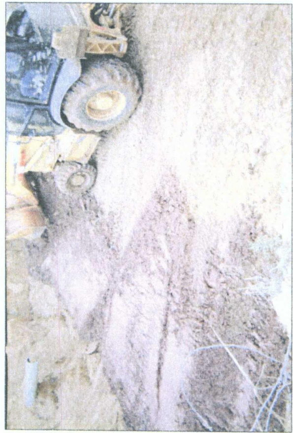
installing clay at 6 ft BGS 8/24/2006
