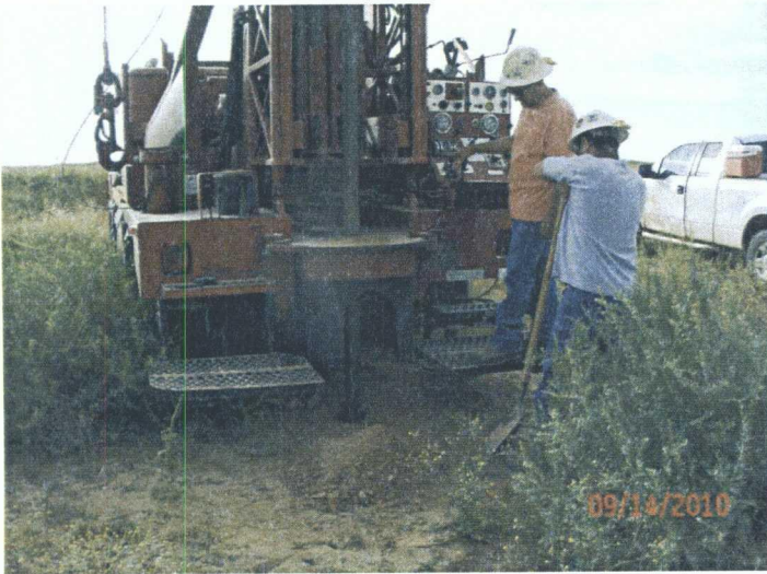
Drilling soil bore #1
